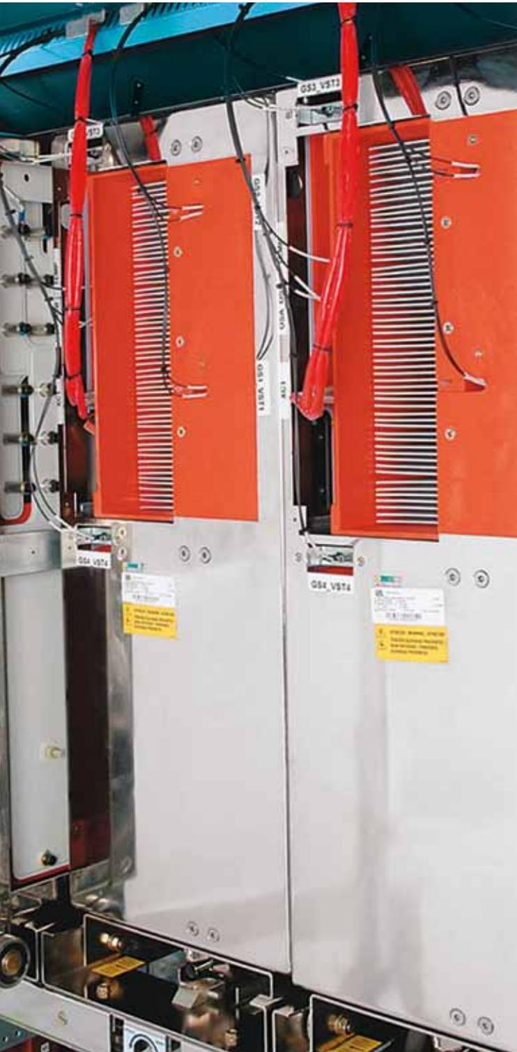
MVW01 follows the same programming philosophy of the WEG low voltage inverter line, simplifying its application. It has a multilevel topology with high-voltage IGBTs (3.3 or 6.5 kV) and optimal switching reducing the motor harmonic currents to extremely low levels. The few number of power component parts, increasing its efficiency and reliability.
